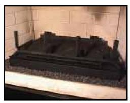
Figure 6 - Placing the Grate Assembly
